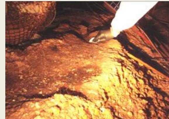
**The commission of dust suppression system had allowed fixing the radioactive dust on surfaces of sub-roofing space of «Shelter» object.**
