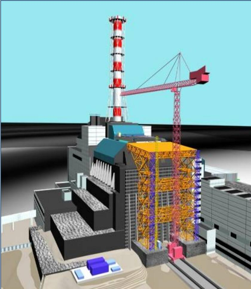
**The works for SO building structures' stabilization were aimed at excluding of probability of potential accidents associated with destruction of building structures and prolonging the lifetime of «Shelter» safe operation ( 15 years ) before the completion of New Safe Confinement erection.**
